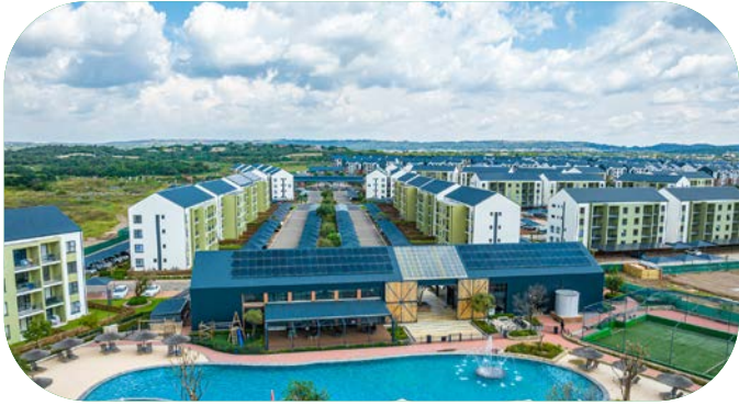
GREENCREEK® HAZELDEAN - TSHWANE
