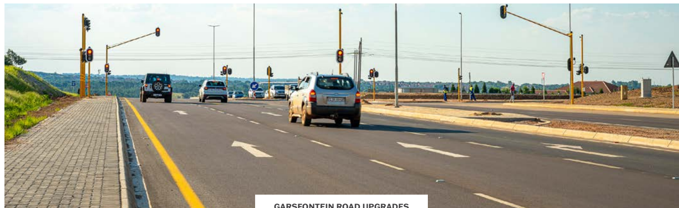
GARSFONTEIN ROAD UPGRADES
