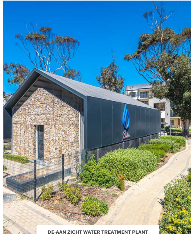
DE-AAN ZICHT WATER TREATMENT PLANT
